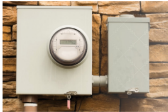
An advanced meter is installed at a home. Source: U.S. DOE. AMI and Customer Systems.
